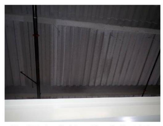
Photo 17: An observable dark area of fireproofing is located at the ceiling of Storage Room 339. Please refer to the infrared image in Photo 17 to view the moisture above the metal decking in this area.
