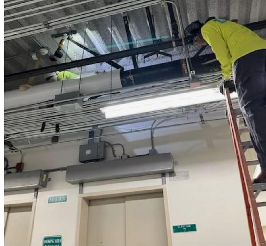
Reinsulating chill water pipes throughout building. Breaks in insulation causing leaks in the Intermediate level service corridor, Main Kitchen and Parking level.
