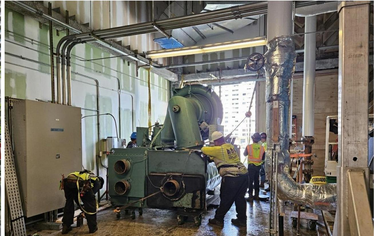
Second crane lift to remove and install remaining two chillers
