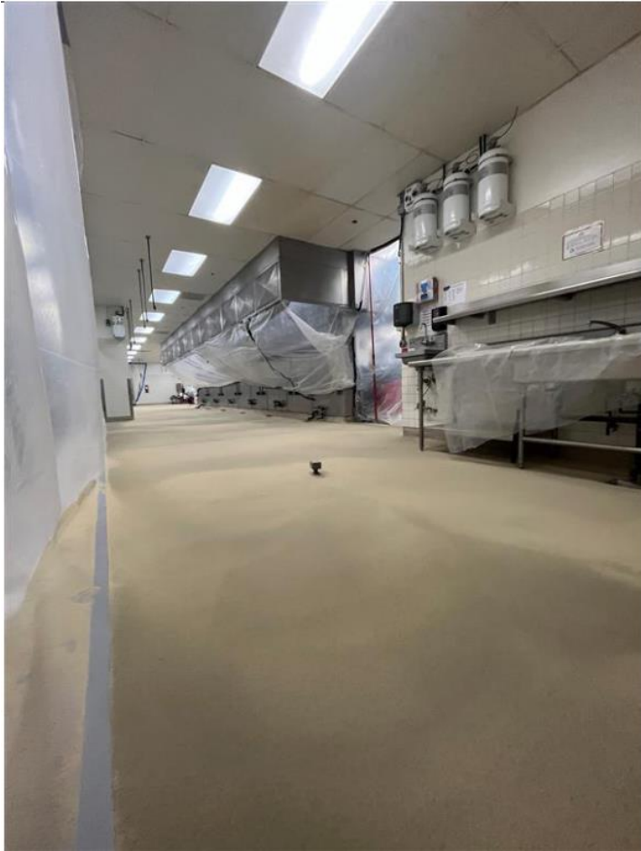
BEFORE: Old flooring
