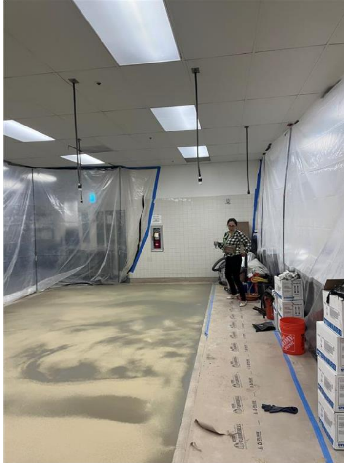
REMOVAL: Flooring preparation
