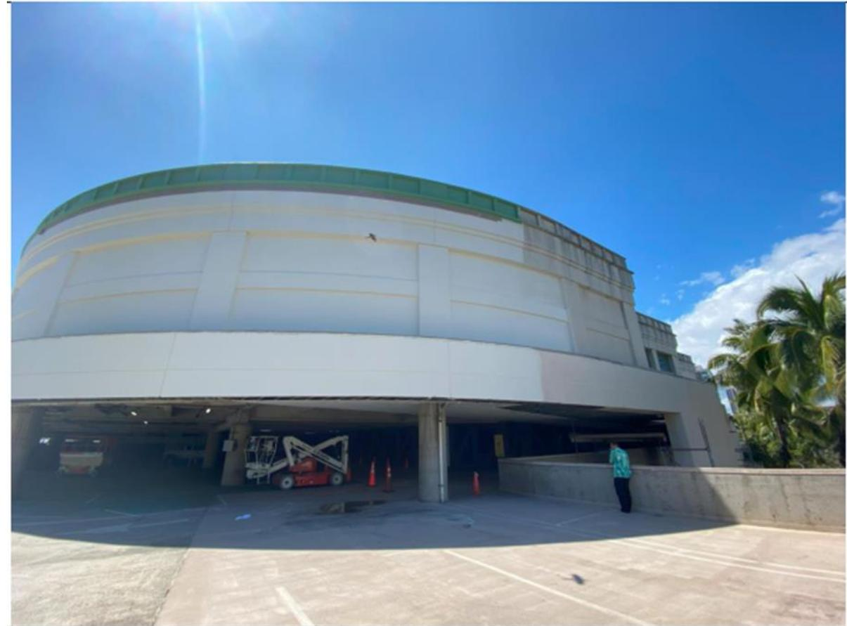
Painters working on the curve around Theatre 310. The Parking deck provides easy access using the boom lifts. Other areas are challenging requiring scaffolding and swing stages.
