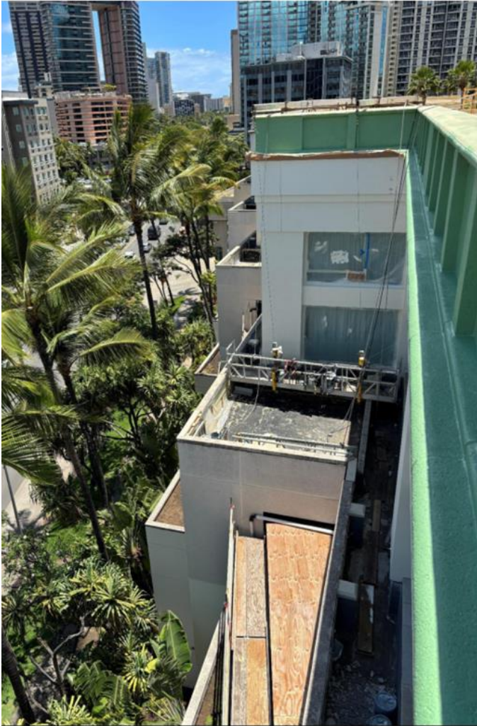
Painters working from swing stages and within planters to access the walls on the Kalakaua Ave side of the building.
