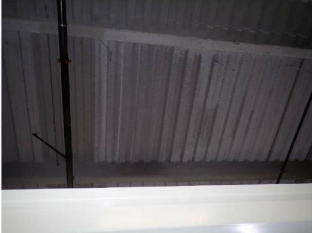
**Photo 17:** An observable dark area of fireproofing is located at the ceiling of Storage Room 339. Please refer to the infrared image in Photo 17 to view the moisture above the metal decking in this area.
